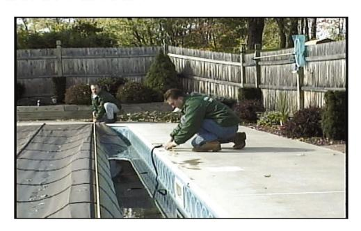
On freeforms cover should be centered over pool using weights on the straps. Again working from the center straps out.
