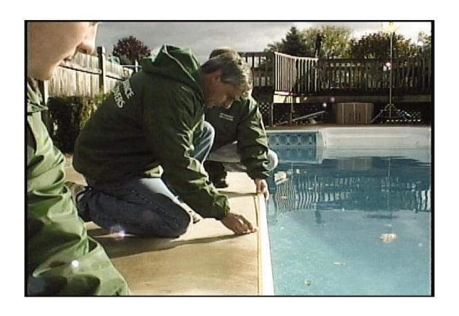
The distance between points is not fixed. It should vary with the complexity of the shape. Closer in tight radii and further apart on straight walls.
