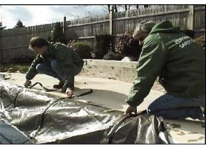
Vacuum holes: To remove dust to ensure depth is open to set anchors.
